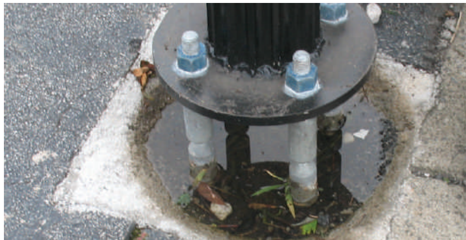
Figure 11. Breakaway footing on a sign post.
